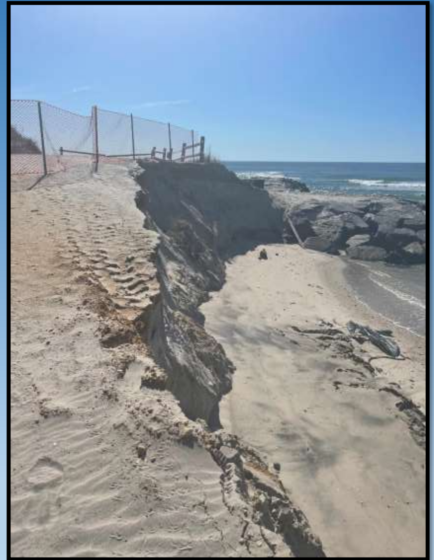
Storm damage from May nor'easter that cut off vehicle access to the beach.
