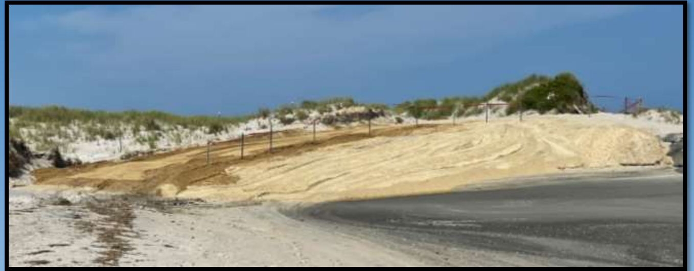
Repaired vehicle access ramp to Stone Harbor Point
